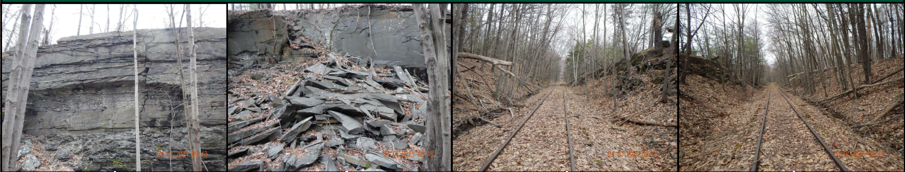
Rock Cut - Approximate Width to Face of Rock 25' - Approximately 3,400 LF
