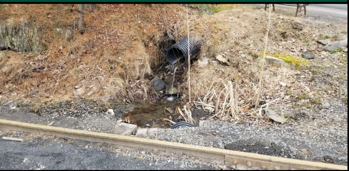
12" HDPE Pipe Culvert
