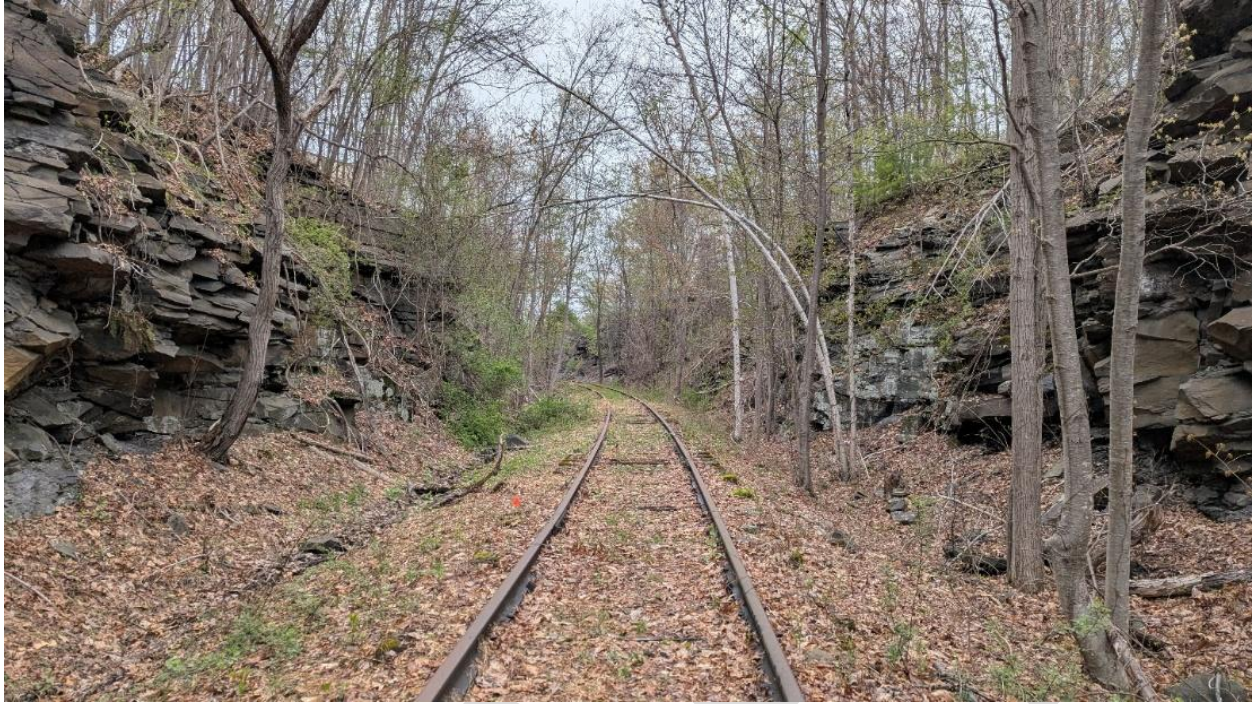
Figure 6 - High Rock Cut Section and Stream Looking West
