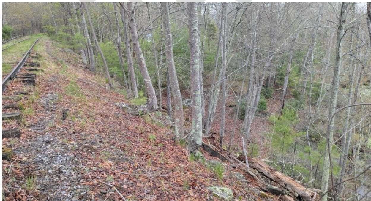
Figure 5 – High Fill Section “Stony Hollow Fill” and Wetland (right)
