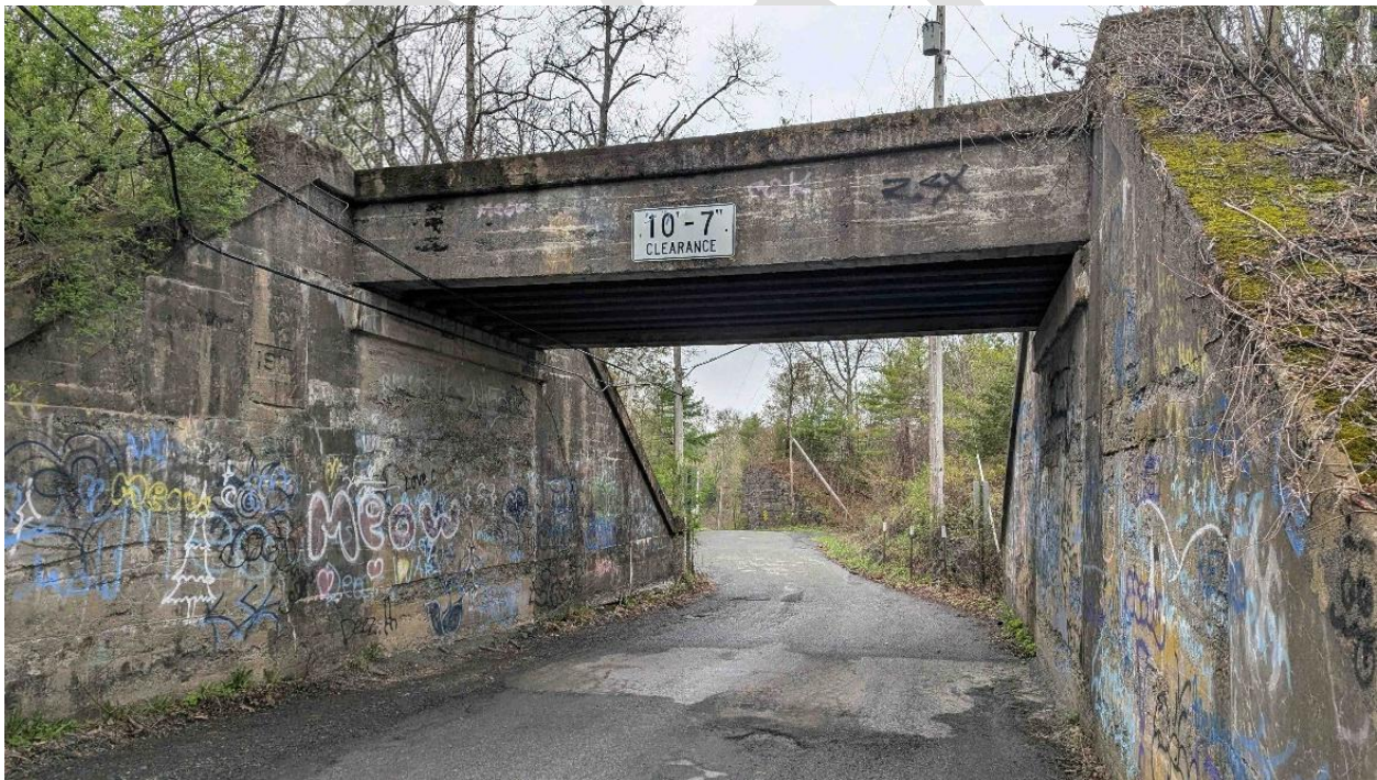
Figure 7 - Beesmer Road Railroad Bridge looking East
